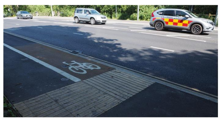
Built in 2020-21, this provides just 1.45m for walking and 1.25m for cycling the latter with no separation from 30mph cars.
